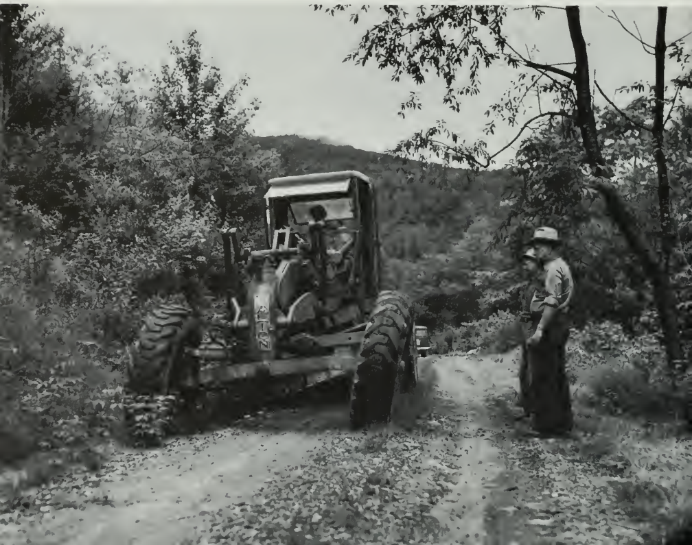
Mr. Seely checks the work of a road maintenance crew.
